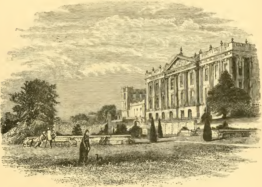
West Front from the South.
